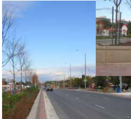
South Gateway streetscape improvements (Main and Steeles)
